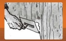
Crack-free plasters of a thickness from 1 mm to 15 mm, produced as a single layer, felted or smoothed. On old, solid substrates for levelling unevennesses, for wet areas, pools, moisture-proof spaces, building socles, water tanks, and plant basins. On concrete, masonry, lightweight concrete, pumice stone concrete, aerated concrete, and lightweight slabs. Protective plaster in case of a missing iron covering.
